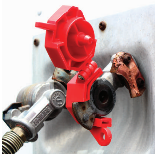
Attach device to Glad Valve.
