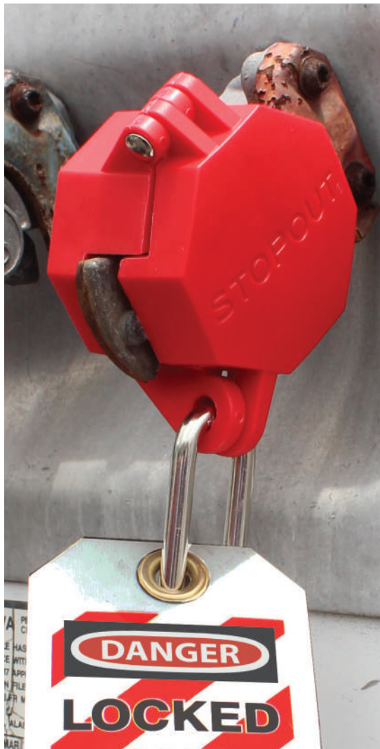
Close device over Glad Valve and secure with padlock (shackle diameter up to 9/32") and tag.
