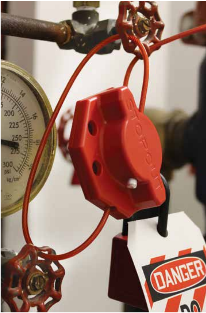
Turn the hasp halves to cinch cable.
