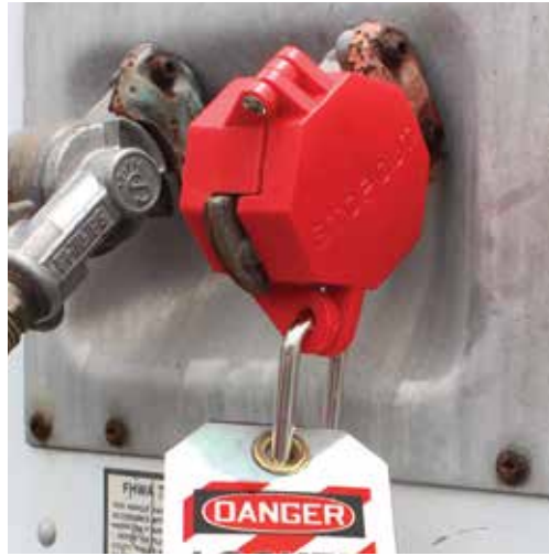
Close device over Glad Valve and secure with padlock and tag.
